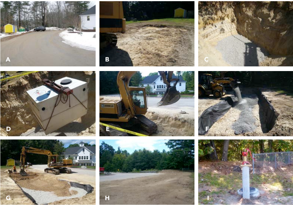
A. Western perimeter drive and parking area; B: re-graded site; C: excavated hole for cistern; D: installed cistern; E: excavated bioretention area; F: placed stone; G: backfilled with BSM; H: finished grade; I: installed cistern pump.
