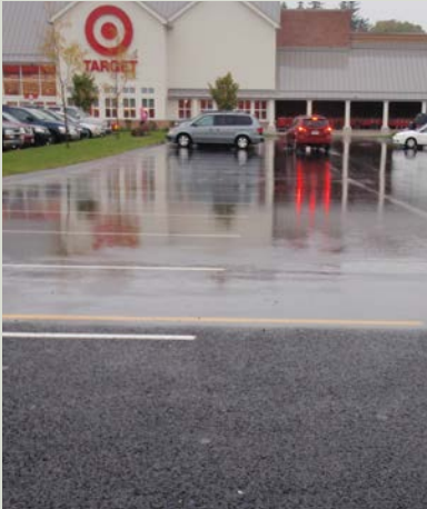
POROUS PAVEMENT STRATHAM, NH
