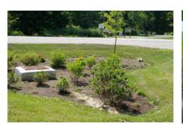
After a heavy storm shortly after construction before the cells were planted, some minor erosion occurred. This demonstrates the importance of site stabilization during or immediately following construction. Use of grass sod on side slopes and on pretreatment filter strips can help to combat erosion in areas with concentrated flow.
