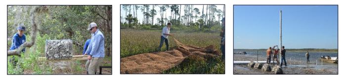
Figure 5: Transporting large gabions (left); coconut fiber mat (center); installing piling (right)
