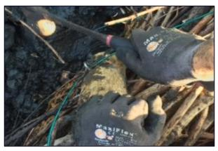
Figure 10: Compressing tree branches and securing with wire to fence post
