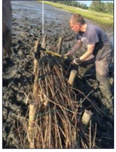
Figure 7: Project team installing fence posts using wood mallets
