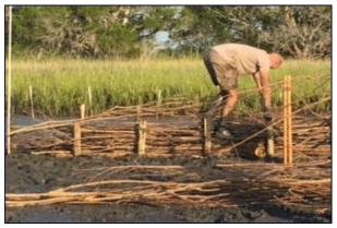
Figure 9: Adding tree branches inside the fence posts and compressing until packed
