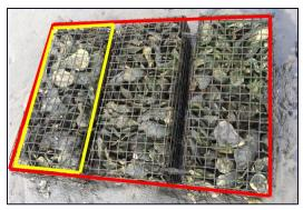
Figure 19: Larger oyster gabion set is outlined in red and small, individual oyster gabion is outlined in yellow
