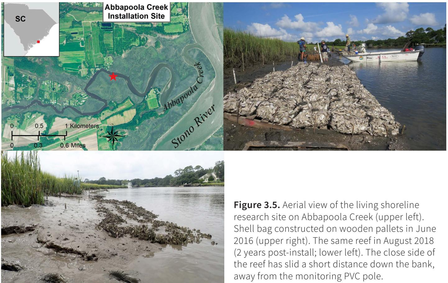
**Figure 3.5.** Aerial view of the living shoreline research site on Abbapoola Creek (upper left). Shell bag constructed on wooden pallets in June 2016 (upper right). The same reef in August 2018 (2 years post-install; lower left). The close side of the reef has slid a short distance down the bank, away from the monitoring PVC pole.
