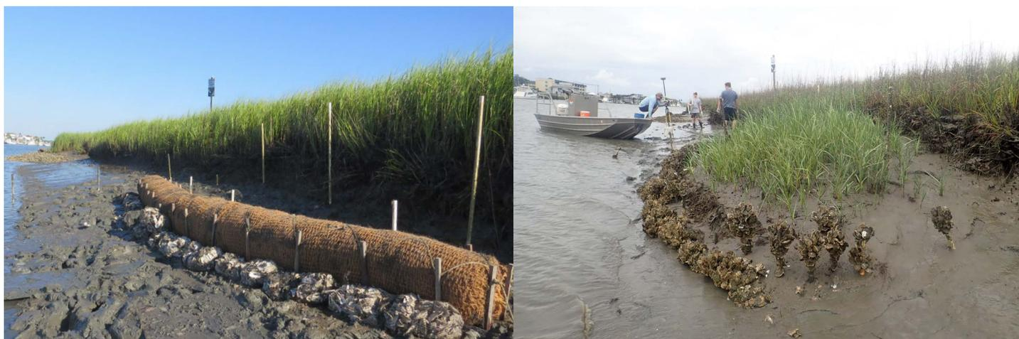
**Figure 5.2.** Single-row coir log treatment with a single row of shell bags, installed in July 2016 along Big Bay Creek (left). This treatment was planted with smooth cordgrass in April 2018 and photographed in May 2019 (right)
