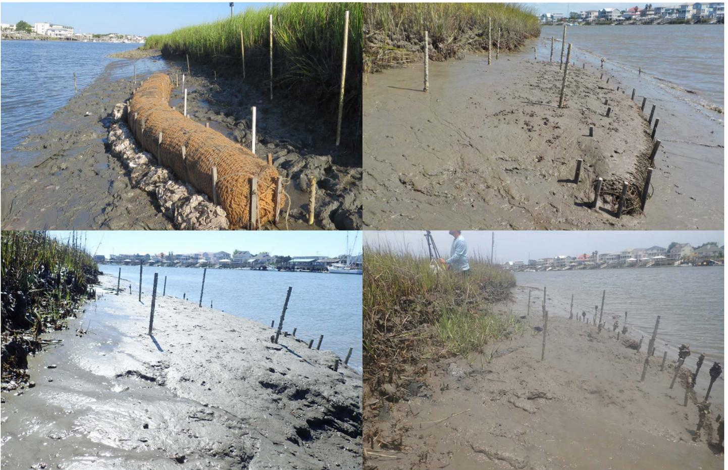
**Figure 3.16.** A single-row coir log treatment at Big Bay Creek (Figure 3.4) in July 2016 (upper left), October 2017 (upper right), September 2018 (lower left), and May 2019 (lower right).
