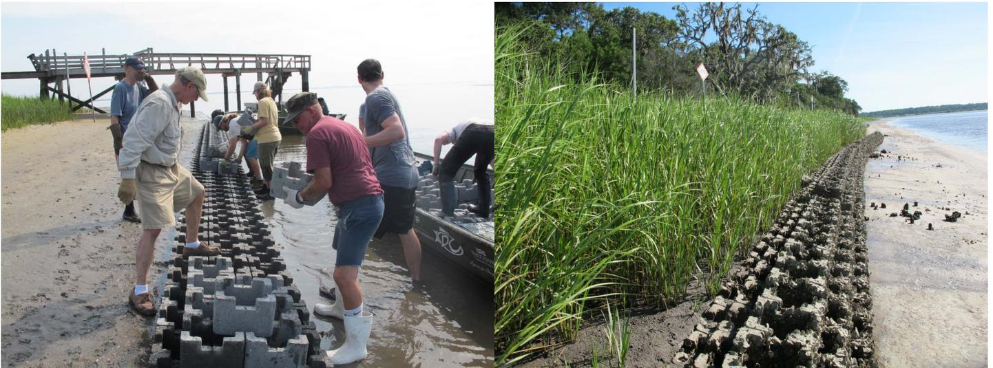
**Figure 3.21.** Oyster castle reef on Lucy Point Creek, near Beaufort, SC, shown during construction (left) and Coosaw River, near Beaufort, SC, shown 2 years after construction (right).
