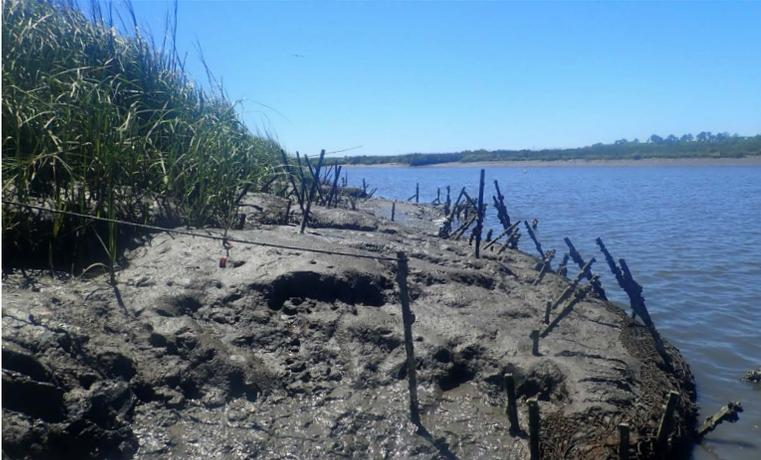
**Figure 3.20.** A double-row coir log treatment at Orangegroove Creek in August 2017 (top). The same coir log treatment in May 2018, with smooth cordgrass freshly planted in the sediment trapped between the logs (middle); full view (bottom left) in April 2019.
