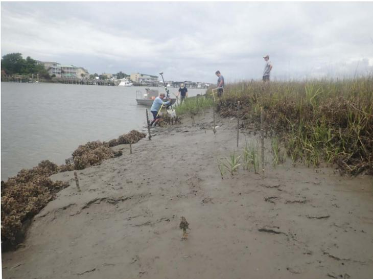
**Figure 3.10.** Almost 3 years after installation of the MWR at Big Bay Creek, oyster cover and growth continue to increase, and marsh expansion was starting to occur. Photo taken in May 2019.
