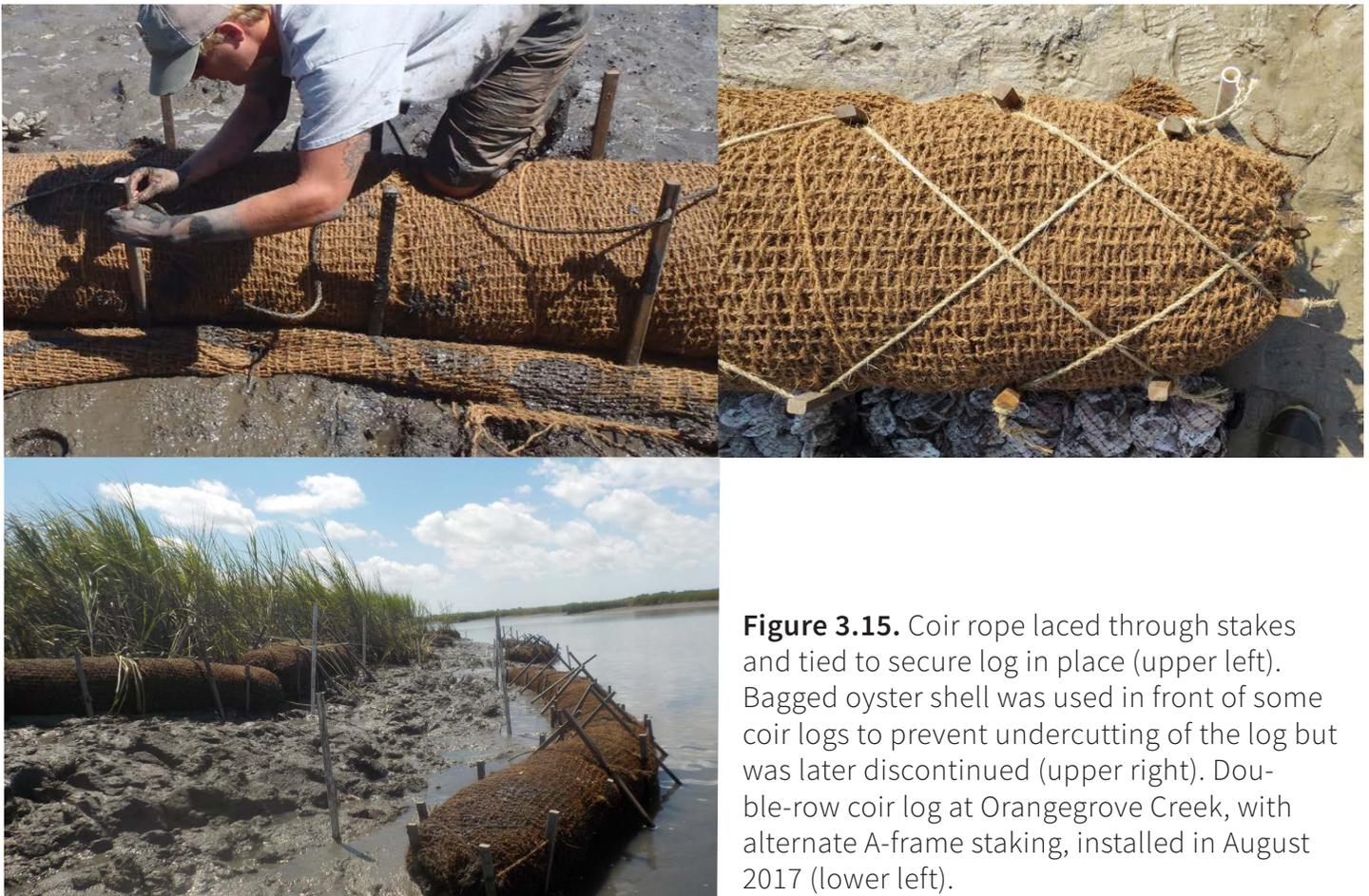
**Figure 3.15.** Coir rope laced through stakes and tied to secure log in place (upper left). Bagged oyster shell was used in front of some coir logs to prevent undercutting of the log but was later discontinued (upper right). Double-row coir log at Orangegrove Creek, with alternate A-frame staking, installed in August 2017 (lower left).
