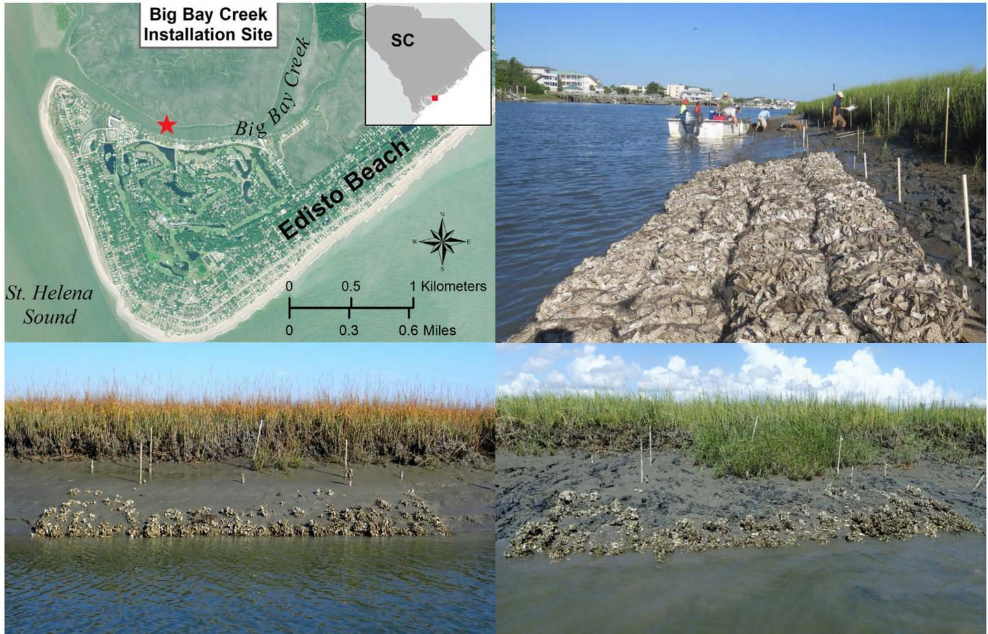
**Figure 3.4.** Aerial view of the living shoreline research site on Big Bay Creek (upper left). Shell bag reef constructed on wooden pallets in July 2016 (upper right). Oyster growth and sediment accumulation on reef at Big Bay Creek in November 2017 (one year post-install; lower left) and in September 2018 (two years post-install; lower right). Note marsh grass expansion (lower right).
