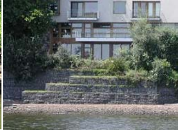
Figure 4: Gabion wall.
