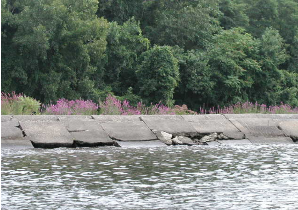
Figure 5: Failing concrete revetment.
