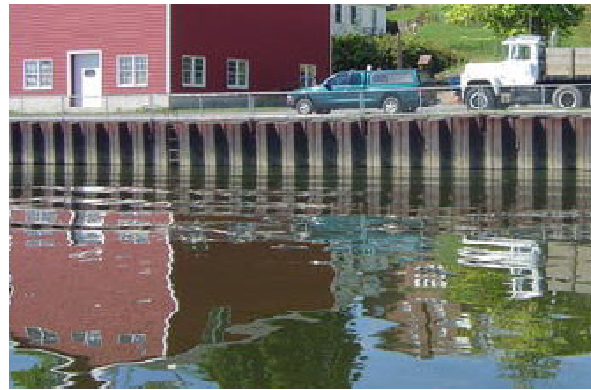
Figure 2: Steel sheetpile bulkhead.
