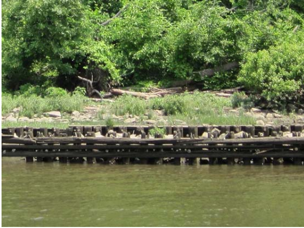
Figure 3: Degraded timber cribbing.
