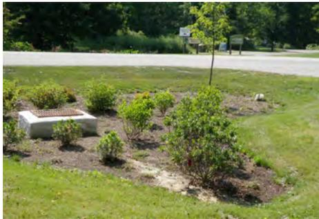
After a heavy storm shortly after construction before the cells were planted, some minor erosion occurred. This demonstrates the importance of site stabilization during or immediately following construction. Use of grass sod on side slopes and on pretreatment filter strips can help to combat erosion in areas with concentrated flow.
